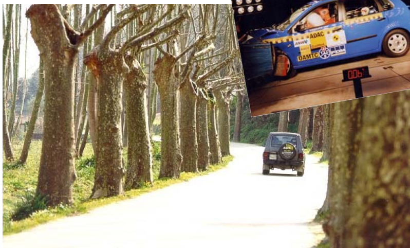
Even 4-star EuroNCAP cars cannot protect against 1-star roads. Unfenced objects at the side of 90 kph roads are a killer. In Germany 1600 die each year striking trees, in France 800 die. Over 500 die striking hazards close to the road in Britain
